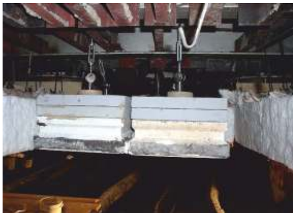
Fig.4: Microporous pre-cast shapes for kiln roof, 400x350x160 mm with high alumina anchor brick and two 50 mm CA-silicate plates on top.
