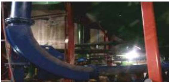
Fig.8 Ejector after installation at site
