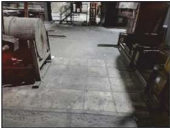
Figure 5: Image of a pre-casted area in the foundry facility in Nagpur prior to installing new flooring
