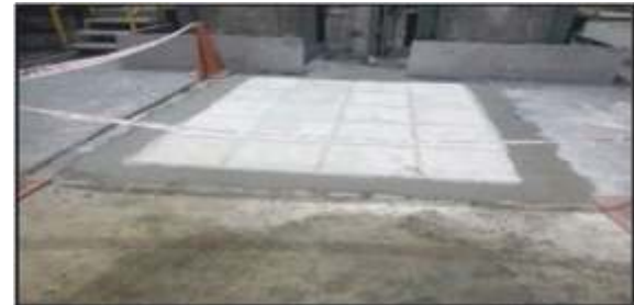
Figure 8: Image of finished section of flooring in Nagpur facility.
