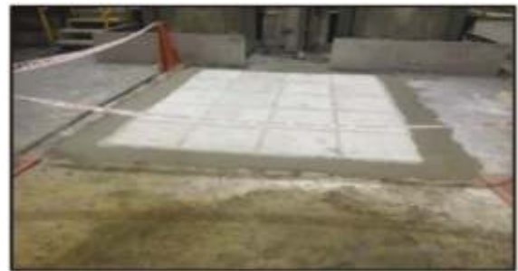
Figure 8: Image of finished section of flooring in Nagpur facility.
